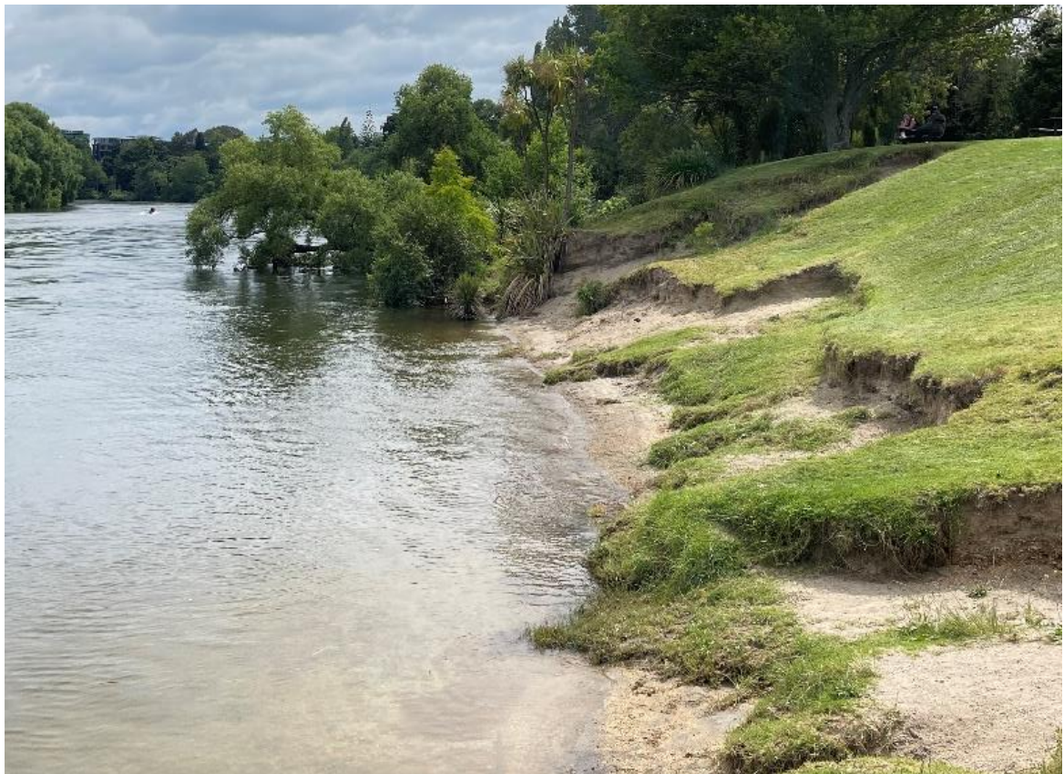
Figure 9. Wellington Street Beach - Unstable banks and vegetation downstream from jetty
