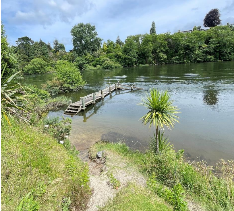
Figure 10. Wellington Street Beach - Debris to east of jetty and sudden drop off
